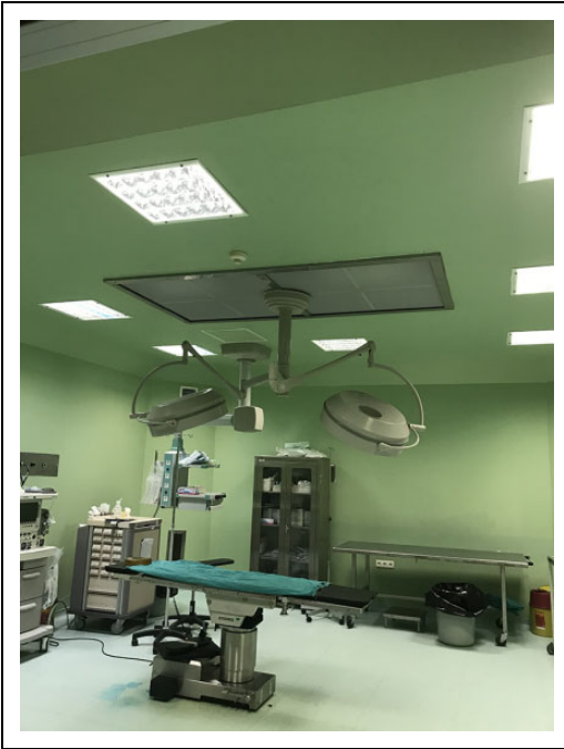
Figure 1. The operating room with laminar airflow systems (LAS-OR).
