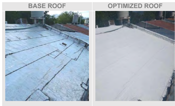
Figure 1. Base roof with aluminum membrane and optimized with smart cladding.
