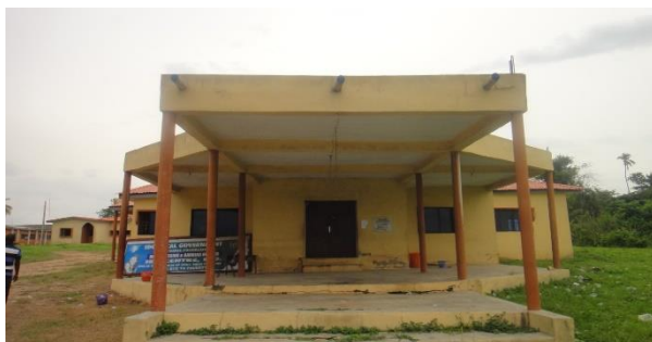
Figure 1: Grasses growing on the crack floors
