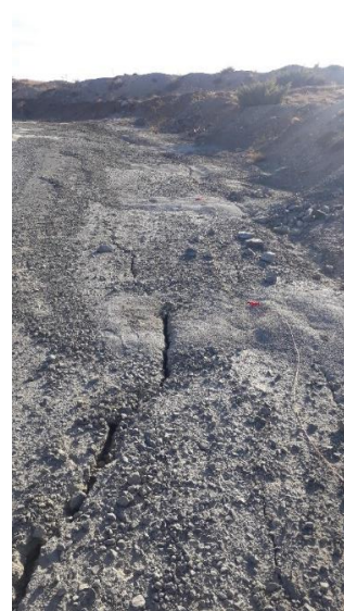
After Blasting (Second Blasting)
