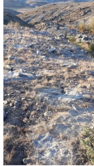
After Blasting (First Blasting)
