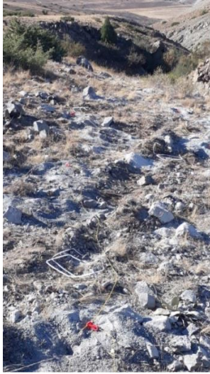
Before Blasting (First Blasting)
