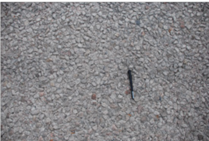
Figure 1. Single layer chip sealed road surface on unbound base layer
