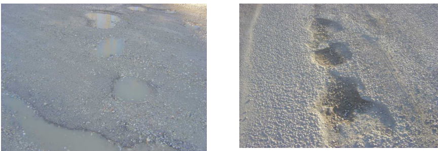
Figure 19. Segregation and fragmentations in chip seals (a and b) (Karaşahin and Gürer, 2007)
