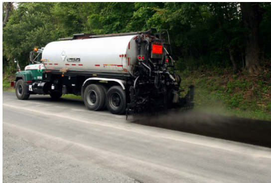
Figure 16. Fog seal application (Reha bitumen 2021)
