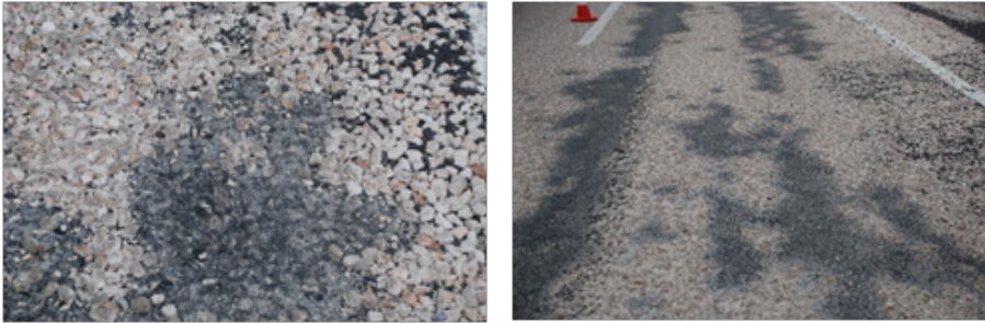
Figure 18. Aggregate raveling on a chip sealed road surface (a) and segregation occurring on the surface (b).
