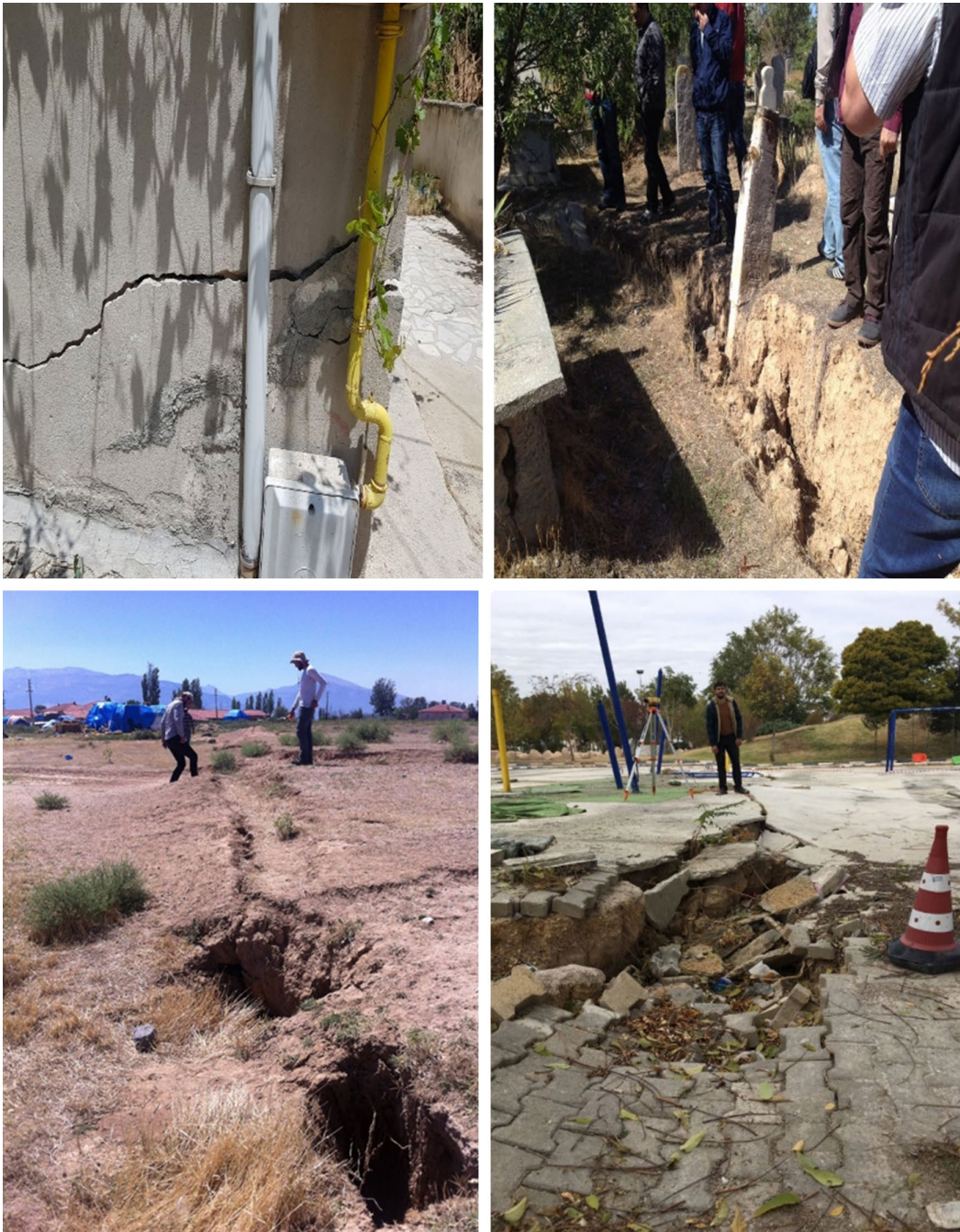
Figure 2. Surface deformations observed in an urban area in Bolvadin.
