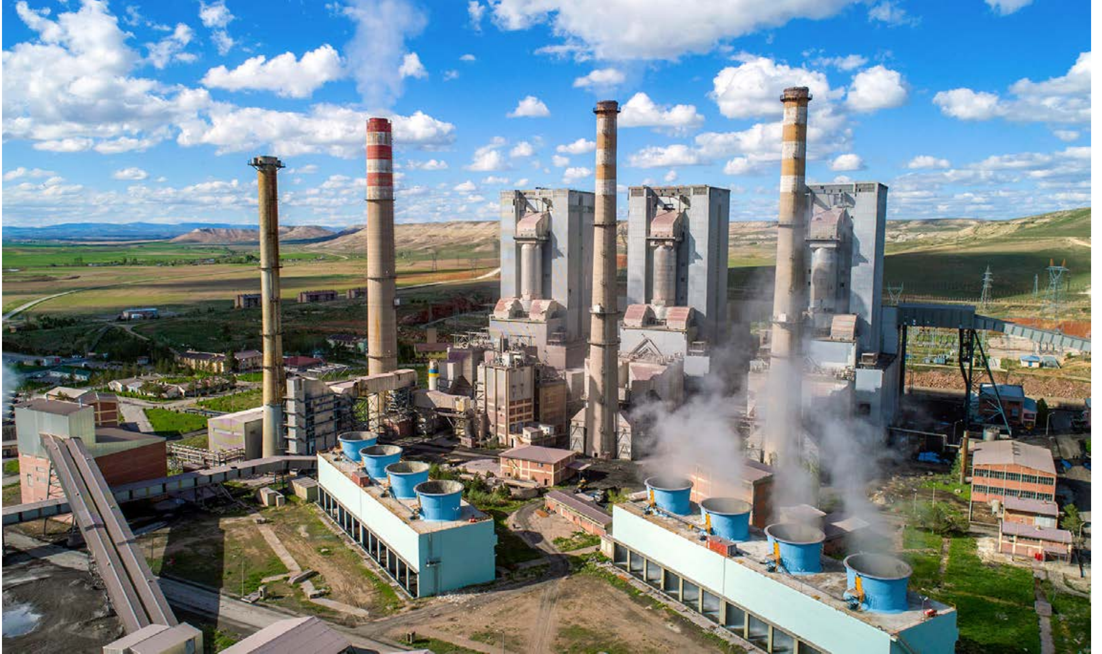
Sivas - Kangal Termik Santrali
