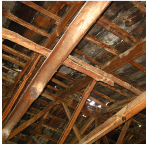
Figure 8. Example of ceiling covering.
