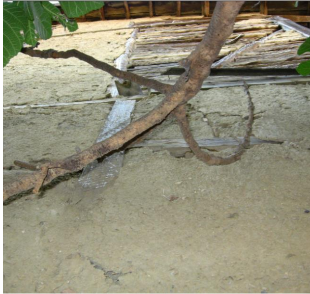
Figure 4. A Mud plastered application example of the facade of the building.
