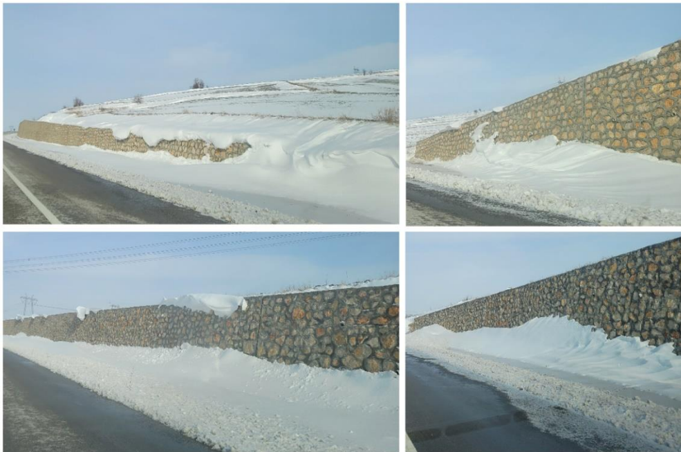
Fig. 6. Photographs of snowdrifts on the water channel and anti-erosion walls due to snowfall and snow plowing from the road on February 6-7, 2023.
