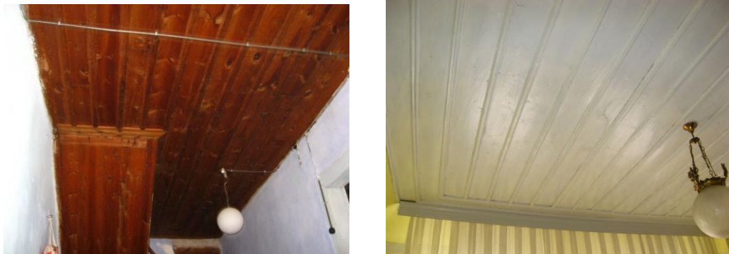
Figure 9. Examples of ceiling covering.
