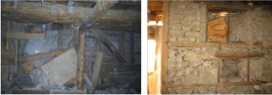
Figure 1. Examples of rubble stone foundation wall.
