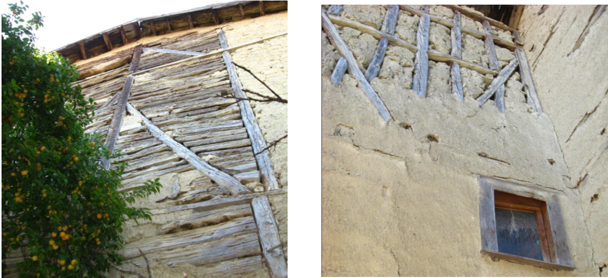
Figure 3. Example of wall detail of wooden structure.
