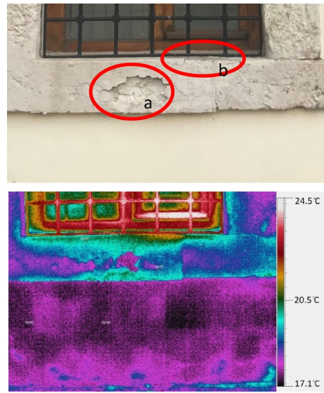
Fig. 16 a Blistering of the limestone window sill; b pores in limestone
