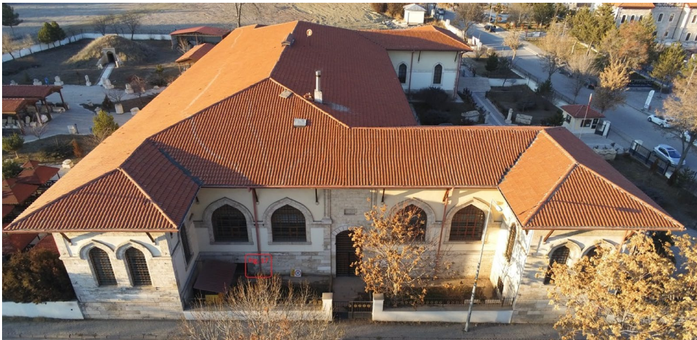
Fig. 9 Southern facade of the Industry School Ironworks Atelier
