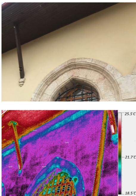
Fig. 12 IRT detection of invisible building materials underneath plaster
